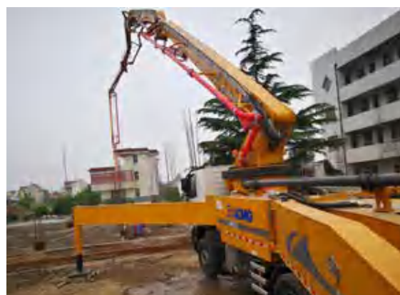
HB52K唐洪工业园区首秀 HB52K boom pump is debuting in Tanghong Industrial Park.
