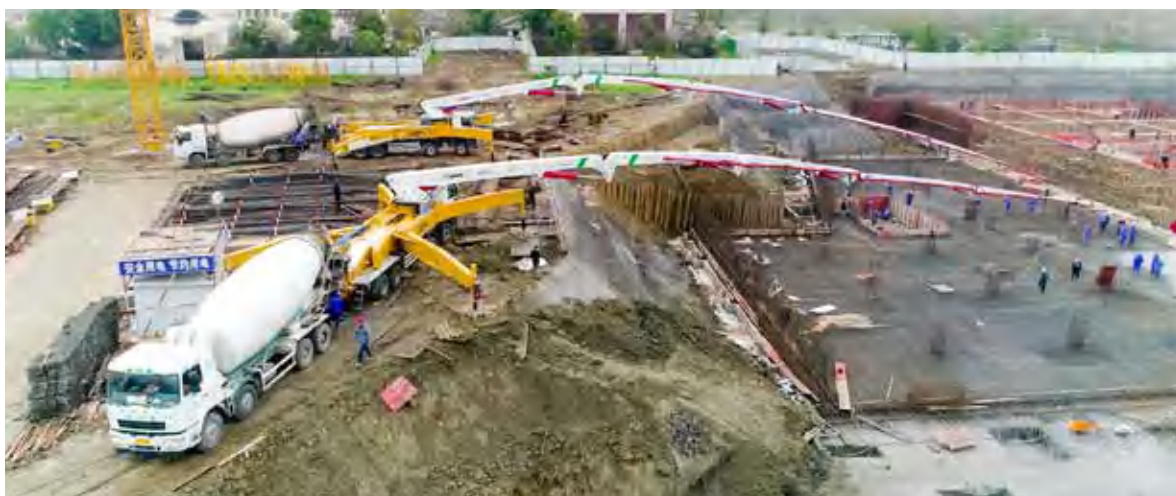
苏州双V7联手施工 Suzhou double V7 teamed up with construction
