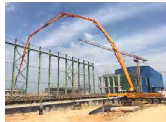
马来西亚第一台HB53K助力关丹产业园 HB53K boom pump is working in Kuantan Industrial Park of Malaysia.
